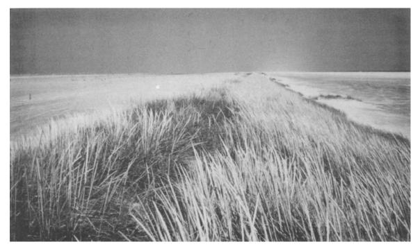
Figure 4-12. Linear shaped, planted dune system, Outer Banks, North Carolina (courtesy of R. P. Savage)
